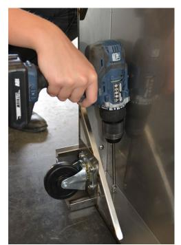
4. With one leg place it on the ground and line up the holes near the wheel and the leg. Use the drill and secure the leg to the wheel base. Each leg will need 4 screws. Replace with other legs.
