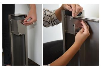
5. Unscrew the screws on the two legs that have the clips. Line up the one of the side panels (table) and secure. Repeat on other side.
